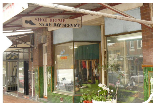
Traditional shop fronts
