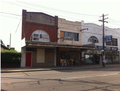
102-108 Canterbury Rd ("Central Buildings")
