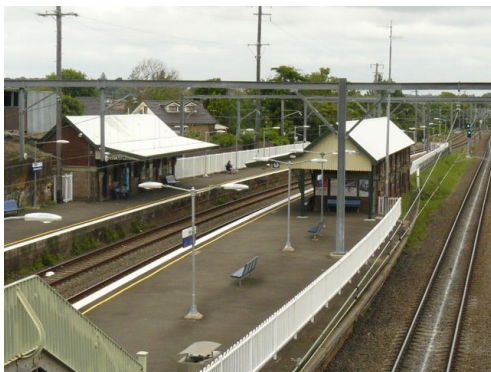
Railway platform buildings
