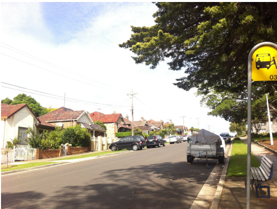
Floss St Street scape facing West
